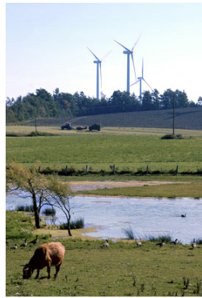
A New York State wind project.
