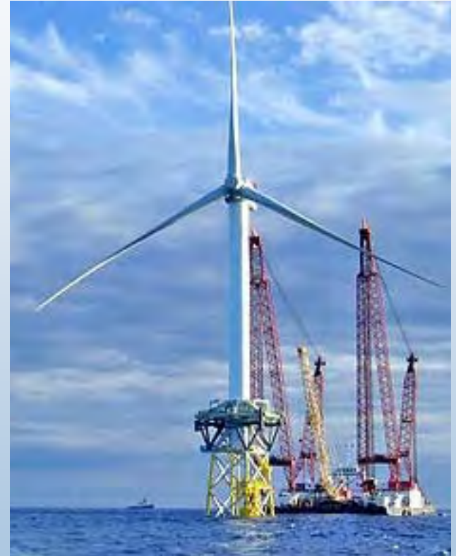
Repower 5MW Demonstration at Beatrice Four-pile jacket
