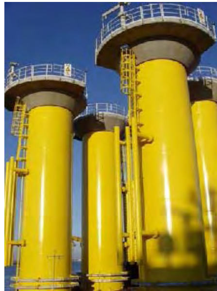
Transition Pieces Credit: DONG Energy
